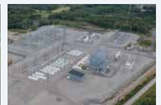
Anttila converter station
